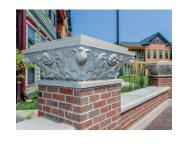
designed this winner in the Unique Architectural Feature category felt cast stone provided the best product and process to successfully reproduce the detail on the historic caps, offering a traditional Indiana limestone look. On-site digital scans of the existing cap were used to create a 3D model, and a rubber mold was created for casting. Judges praised the "very detailed and well executed column caps" and said, "The difficulty of replicating from natural stone to cast stone was impressive."
