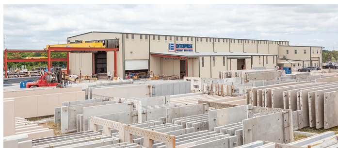
Enterprise’s Corsicana, TX plant was the site of DCS’ first-ever remote installation of its automated liquid color system.
